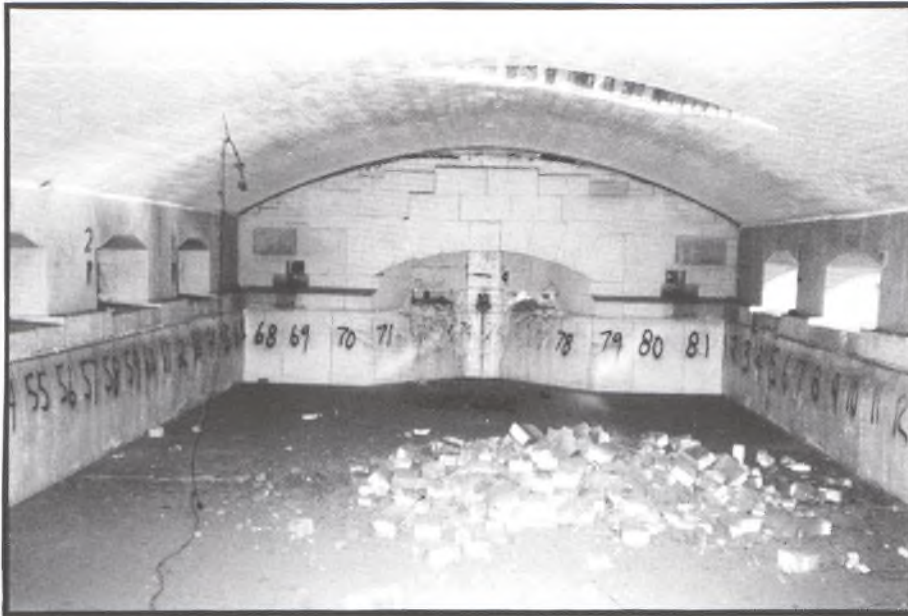
27. North end. (Compare to #5) May 1997 (Courtesy of Bob Stahr)
