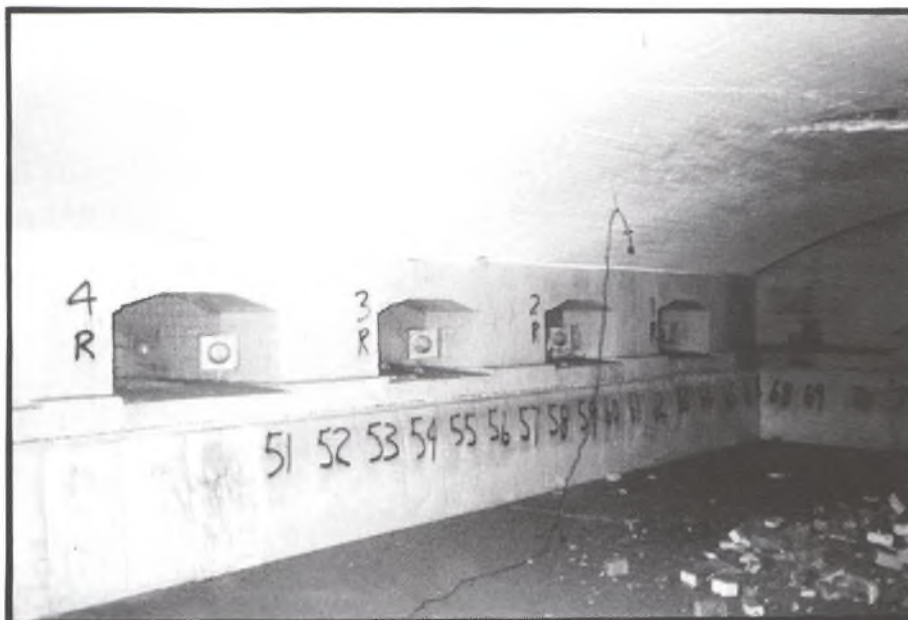
28. West side looking north. (Compare to #16) May 1997 (Courtesy of Bob Stahr)
