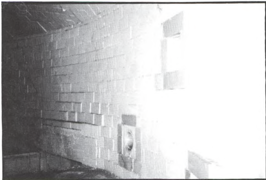
30. Semi-circular section (refining chamber). Lower left corner of photo shows where the glass went out into the feeders and to the molds. May 1997 (Courtesy of Bob Stahr)
