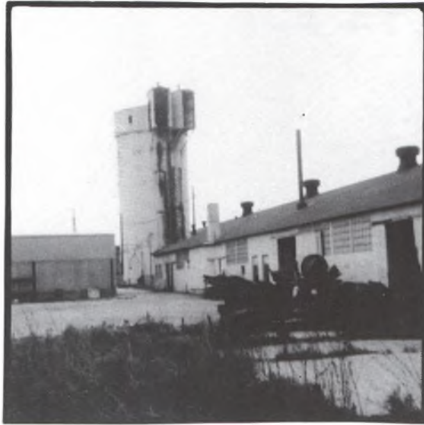
Raw materials silo with warehouse on right. Looking west northwest. 19 May 1981
