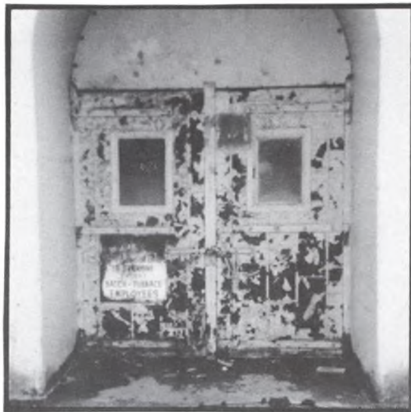
Doors into batch mixer by raw materials silo. Looking north. 19 May 1981
